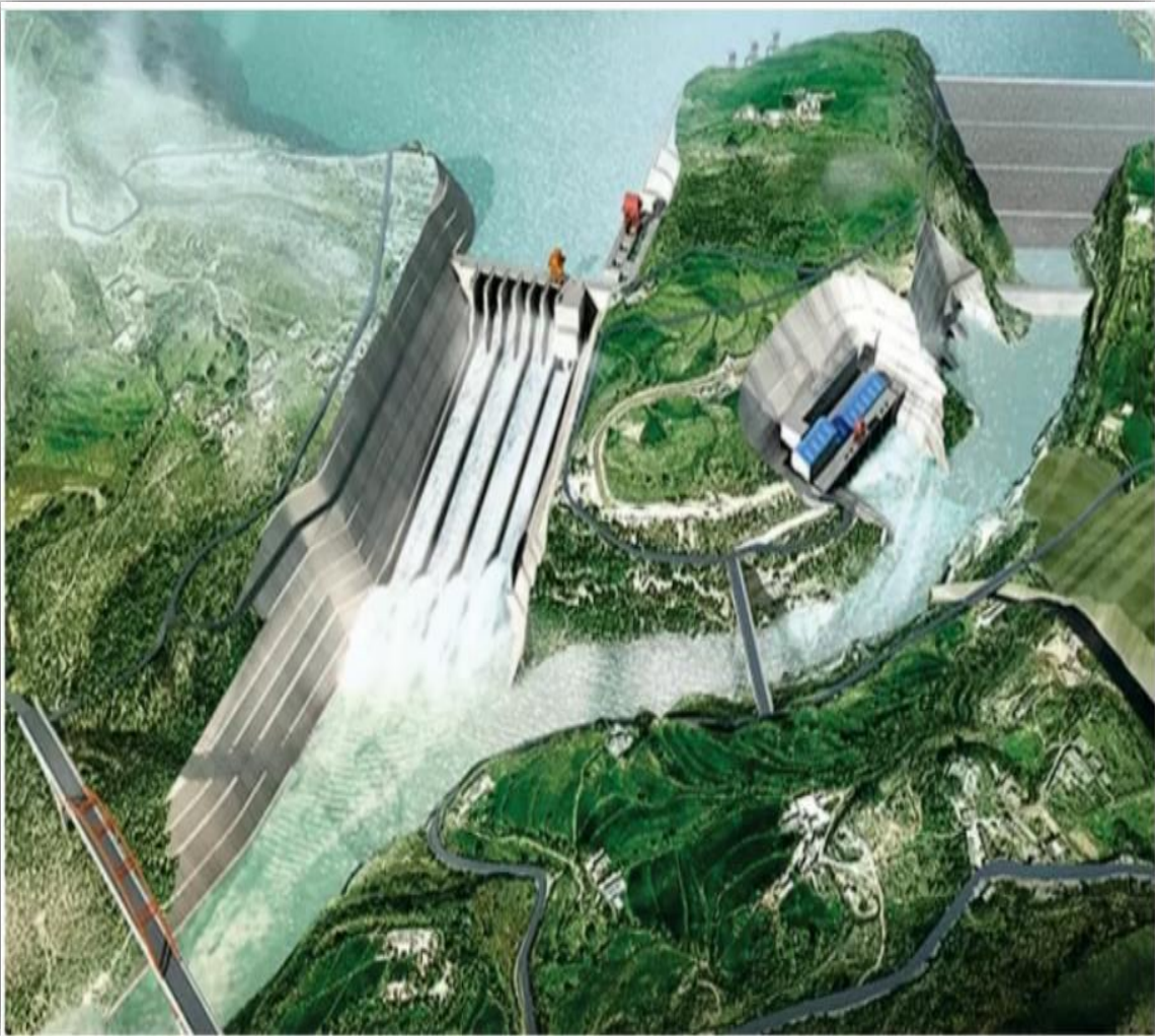
Karot hydropower project
