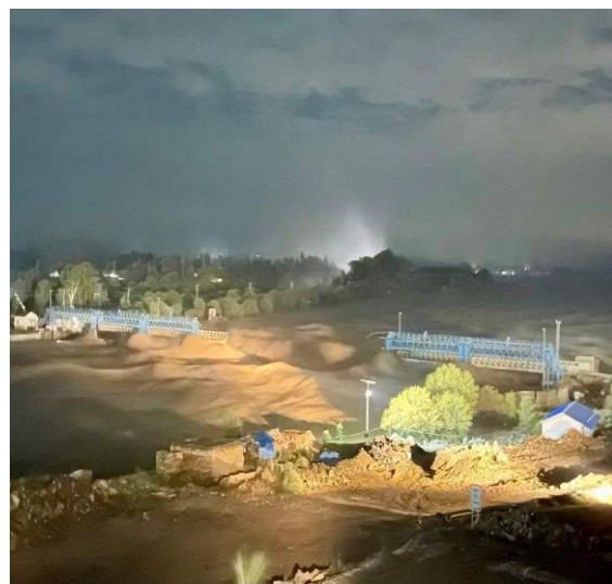
Munda Head Works collapse during 2022 Floods
